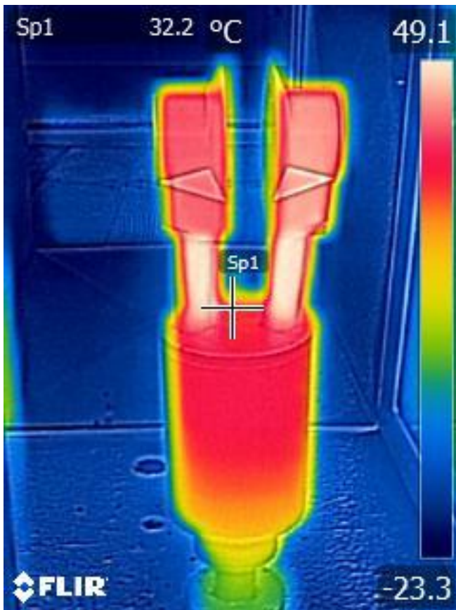
Fig. 7 A thermal camera image of the sensor inside an icing wind tunnel while anti-icing heating is active.
