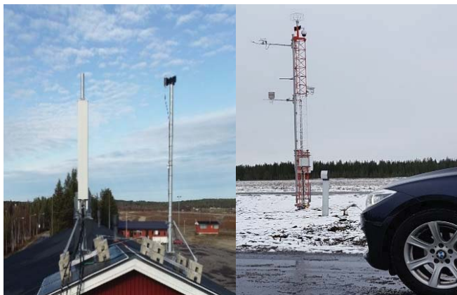
Fig. 5. 5G Test Network and RWS on test track
