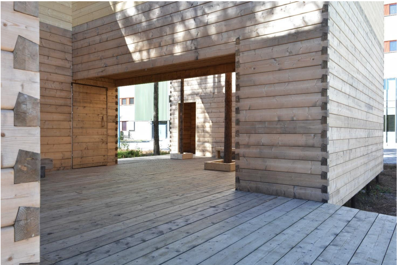
Figure 3. Log structure of the pavilion. [Matti Lakkala]
